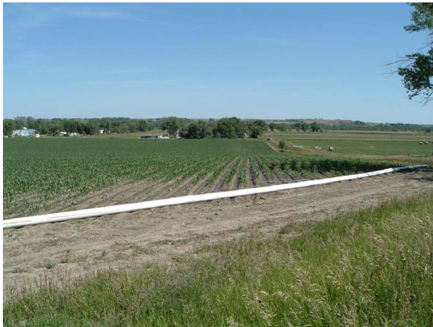
Figure 4. Irrigation Pipeline Delivering Water From the Belle Fourche Irrigation District System to a Field.
