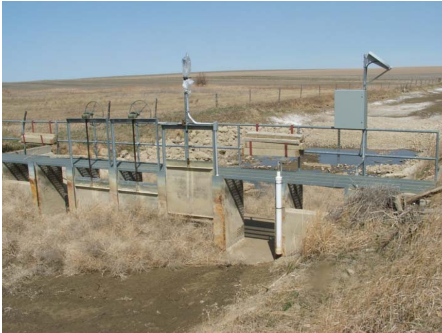
Figure 3. Townsite Check Structure Flow Automation Unit.
